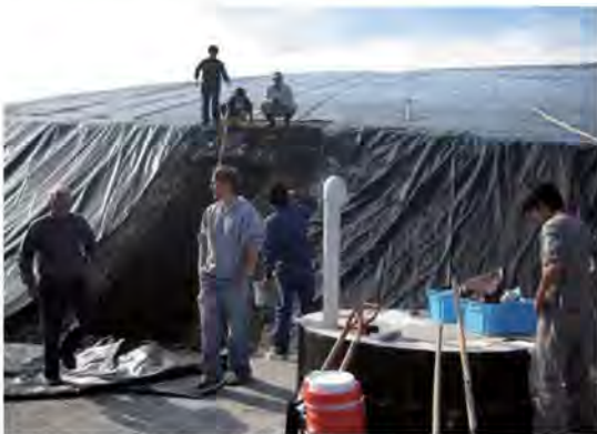
Working at Franklin landfill field
