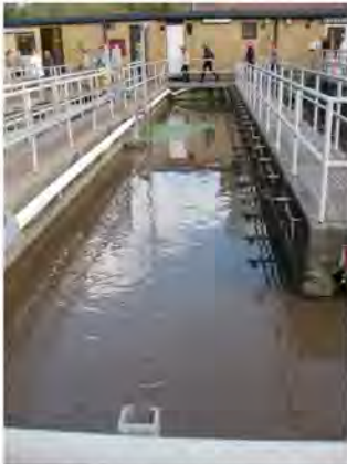
Practical training for analysis of sewage treatment facility
